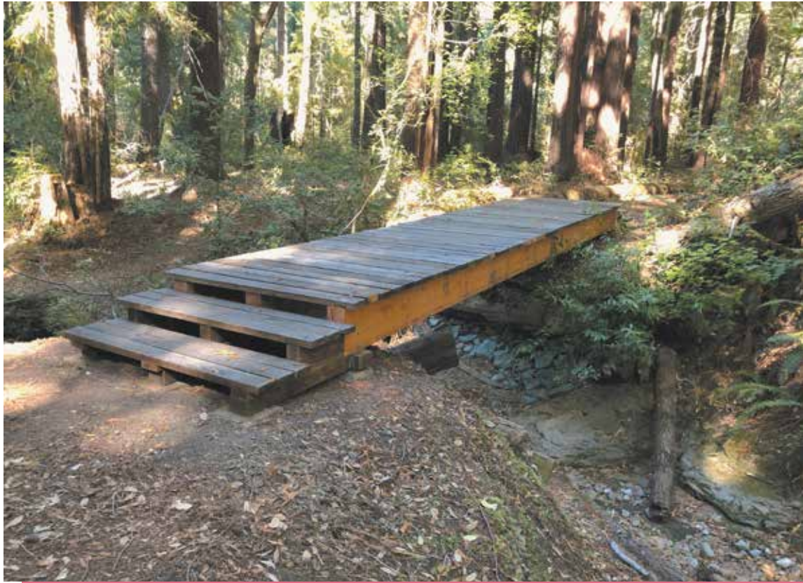
The completed bridge rebuilt by volunteers with The Women's Forest Sanctuary
