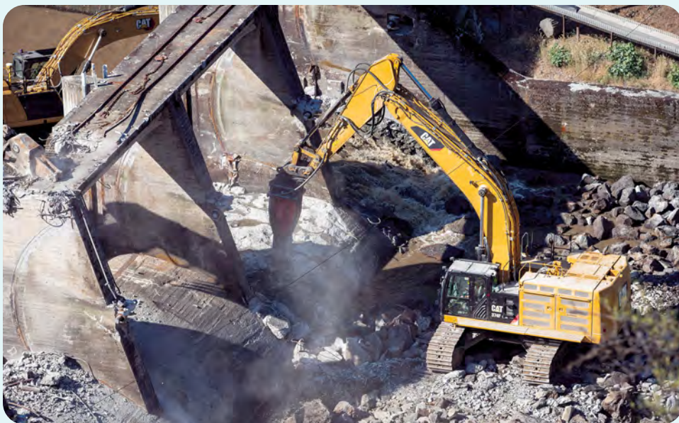
The Copco Dam No. 2 during deconstruction. To see more photos of the before, during, and after removal: https://tinyurl.com/CopcoDam2Photos PHOTO BY SHANE ANDERSON OF SWIFTWATER FILMS
