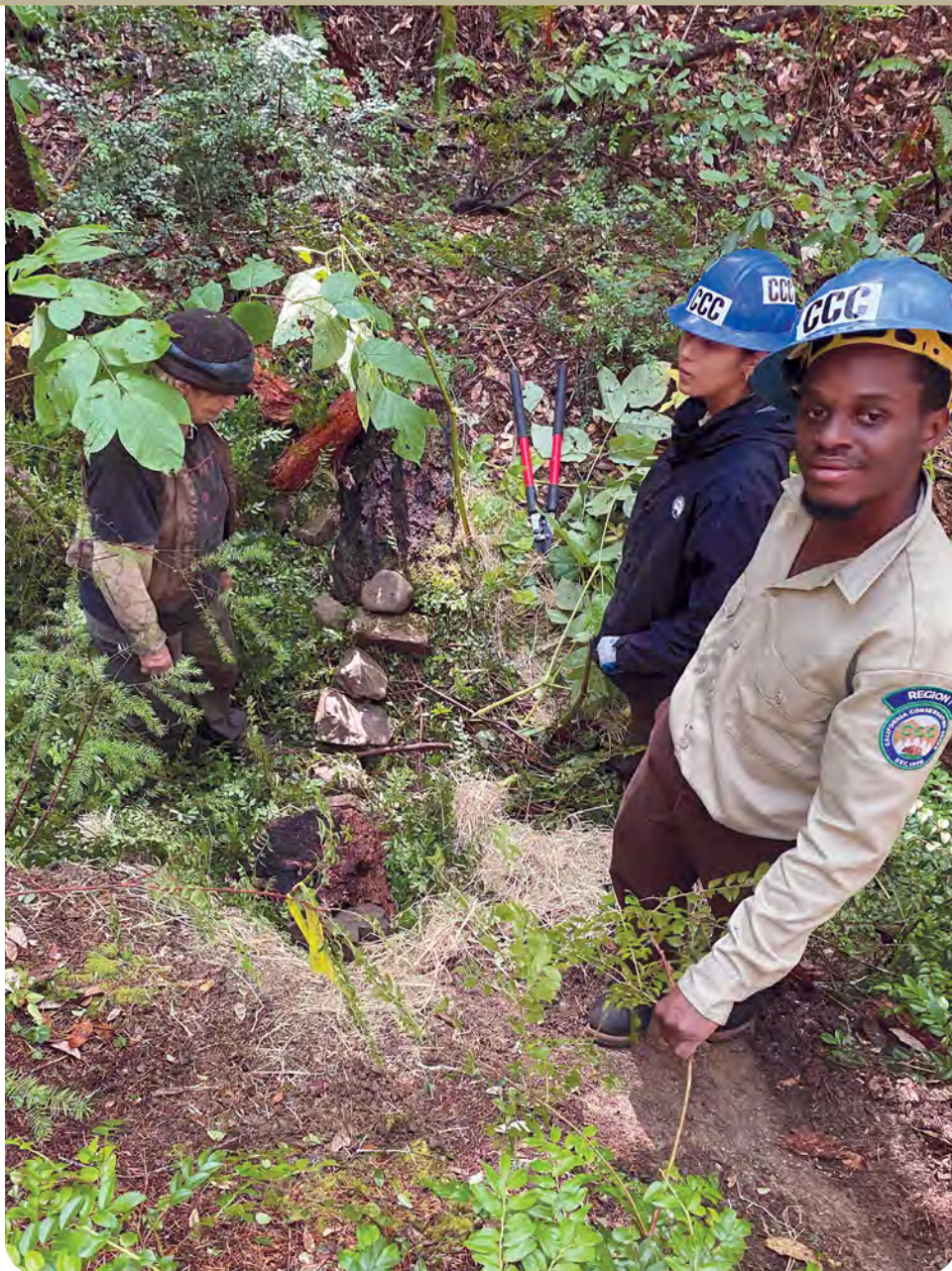
Two CCC members assist as community volunteer, Georje Holper (left), demonstrates for the crew how to branch-pack an incised tributary to McKee Creek.
