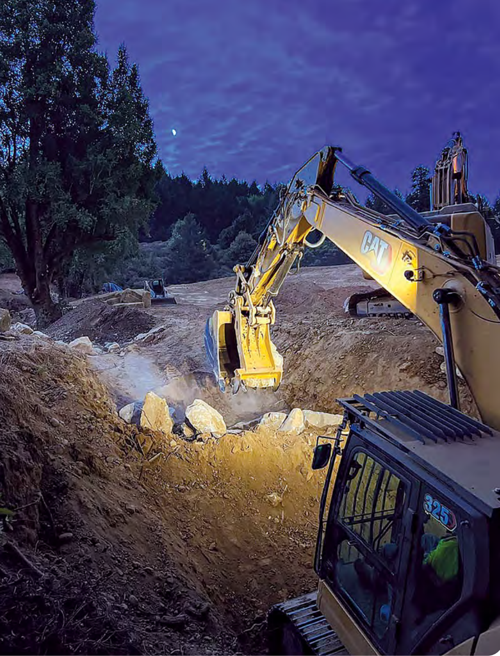
Creating grade control structures on the cooling gallery. PHOTO BY JOAQUIN COURTEMANCHE
