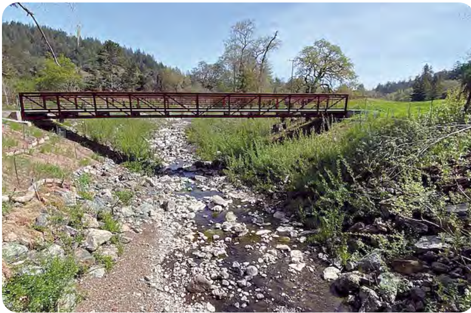
Roy's Riffles restoration site: thick growing willows provide good shade for understory plants.
