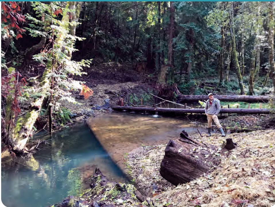
A completed log weir (left) and beaver dam analog (right) in the South Fork of Lost River.
