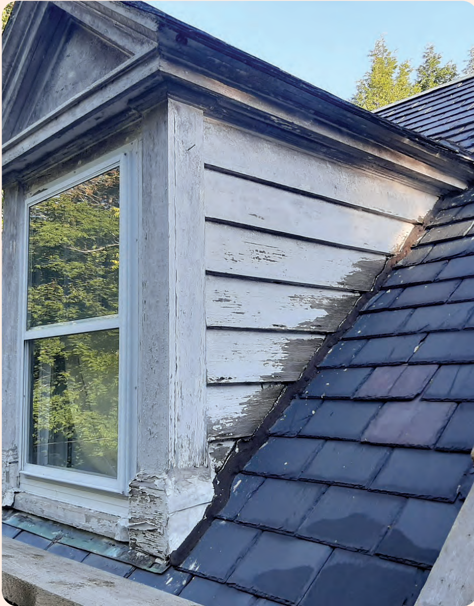
Roof-to-wall intersections are especially susceptible to accumulating debris and moisture, causing rot, which is more combustible than material in good condition. Ensure your roof is constructed properly with at least 6-inch metal flashing along the walls and is kept clean. Good roof care is important all year round! PHOTO SOURCE: HTTPS://JOEGOODEROOFING.COM/WOOD-GUTTERS/
