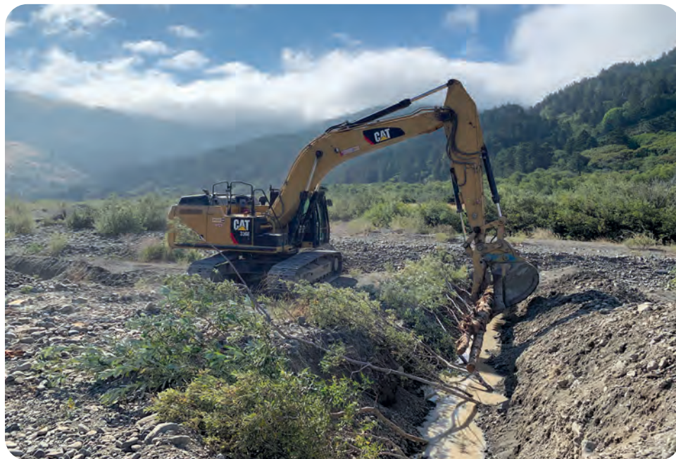
Edwards Excavation and Restoration places wood in a willow baffle.
