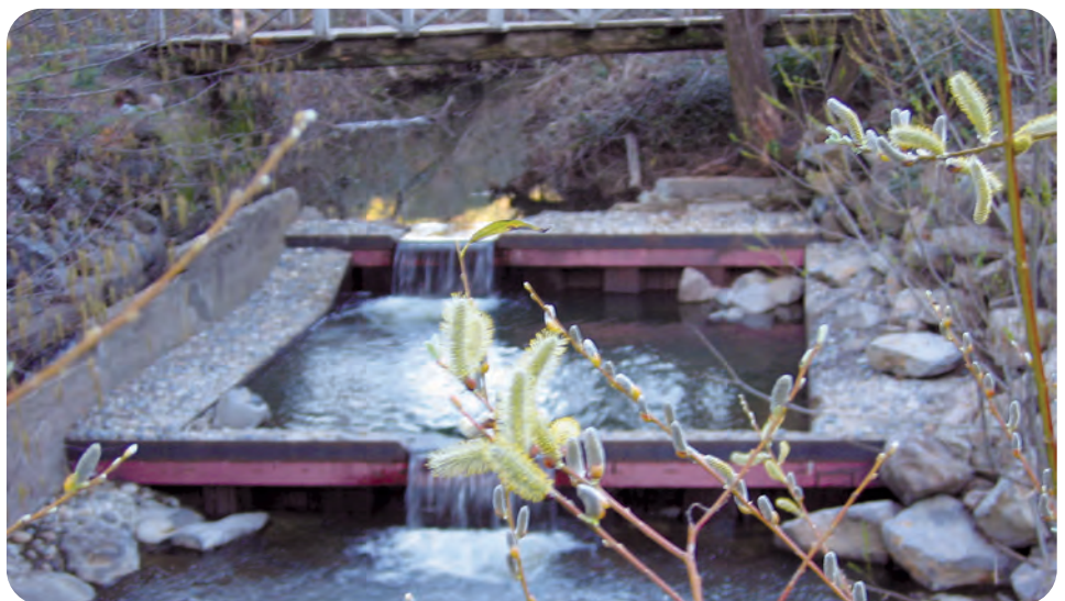
The Roy's Pools structure was a temporary fix installed in 1999 to help fish get over Roy's Dam. While it allowed adult fish passage, it was a trap for juvenile salmonids who became stranded in the spring when water levels fell.
