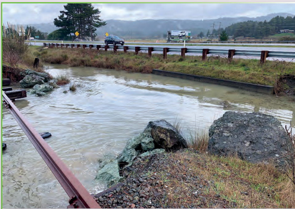
The old railroad dike is all that stands between Highway 101 and Humboldt Bay. Just south of Arcata, a large gap has formed where the King Tides erode the dike with each passing year.
