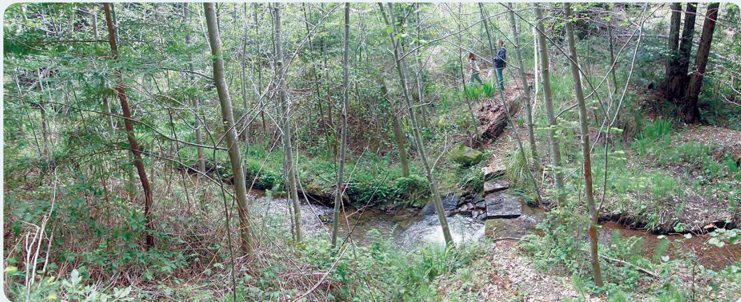
A recovering section of Ancestor Creek that was once a very damaging stream crossing of the main haul road. Ancestor Creek is a coho refugia in the headwaters of the Mattole River. This grade control log structure creates pool habituate and helps to stabilize the creek upstream. Just out of the top of the photo is a ridge that was augmented by the 1000's of cubic yards of soil removed from Ancestor Creek and planted by Mattole Valley Redwood seedlings. Organizations involved included, but not limited to: Mattole Restoration Council, Mattole, Salmon Group, Sanctuary Forest, and featuring exceptional work by Macky McCullough and his crew.
