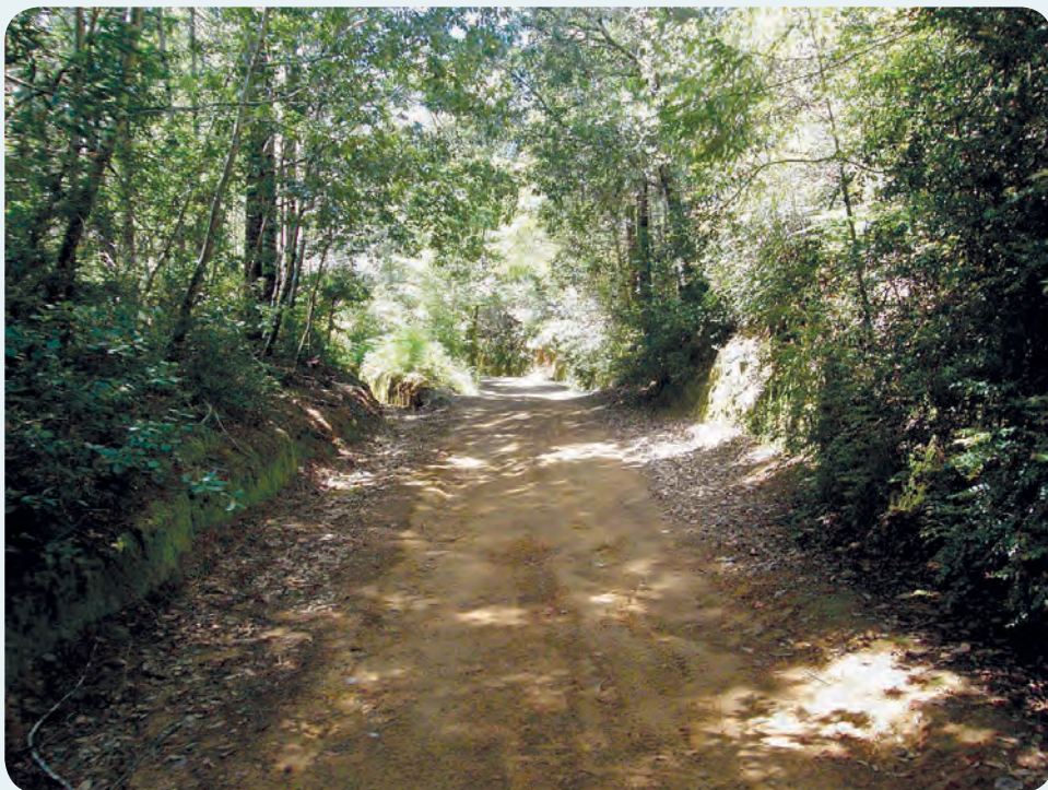
Same portion of road from photo above after repairs about five years ago by a concentrated team effort on about a mile and a half of the worst sections of Usal Road in Waterfall Gulch. The county, so far, has done timely maintenance! The by-pass road, shown in photo above, was closed off and replaced by proper road drainage directing water off of the road with a rolling dip. Other measures used here, and at many other locations, included heavy rocking and careful sculpting of the road surface to prevent sediment from entering the creek and meeting public safety needs. No more quagmire parties or nightmares here. ALL PHOTOS THIS ARTICLE BY RICHARD GIENGER
