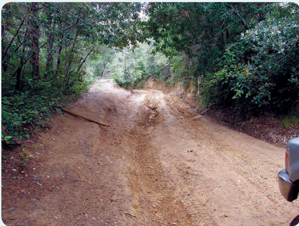
The start of a long existent quagmire on a notoriously erosive and stream-impacting portion of Usal Road, Waterfall Gulch. Sediment generated from this road has directly impacted endangered coho habitat in the North Fork Usal Creek. Note the upper portion of the road on the left that was built by desperate motorists to by pass the quagmire.
